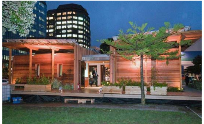
'First Light' eco-house at Frank Kitts Park, Wellington
